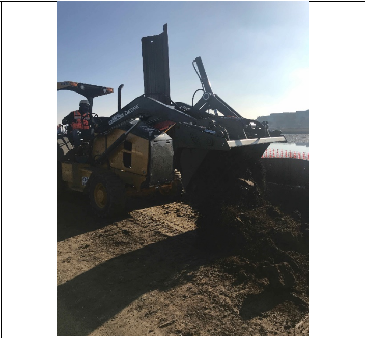
Subgrade preparation near Area 36
