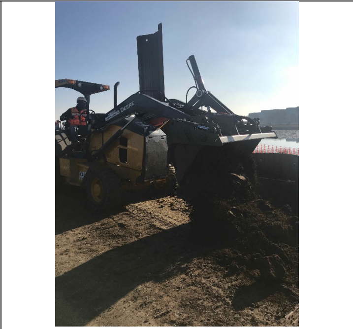
Subgrade preparation near Area 36
